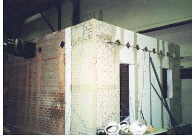
Figure 7 URM repaired with Tyfo materials (strips and web)
