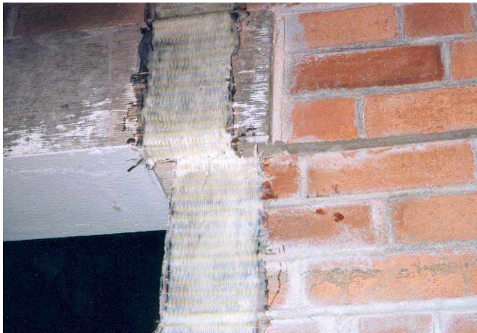
Figure 10 Tyfo strip failed in shear
